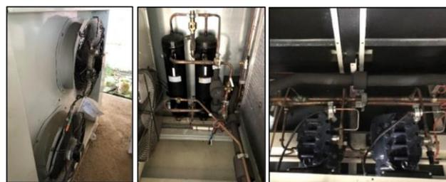
Pictures of the major components installed in the system (Receivers, Condenser fan, Compressors).
